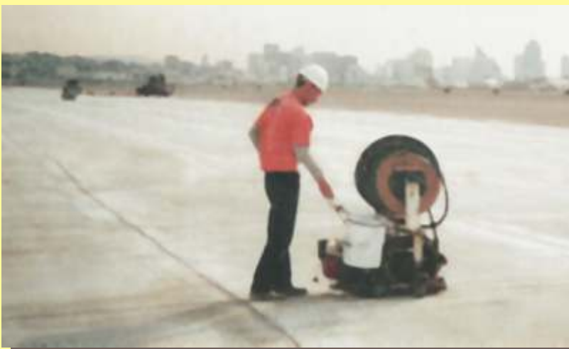
▲ Delastic® Pavement seal application with auto-installer
