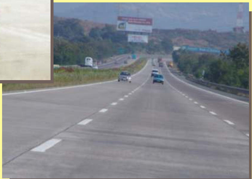
Delastic® Pavement seal application at Mumbai Pune Express Highway ▶
