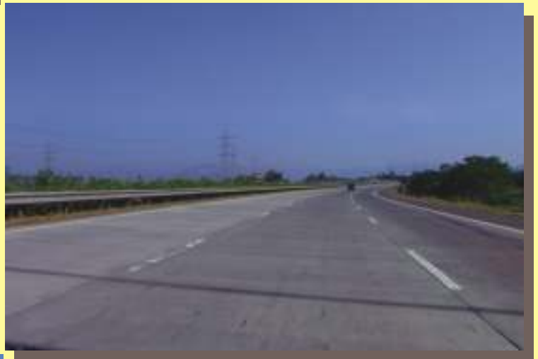
Mumbai-Pune Express highway Elastic - Pavement seal application ▼
